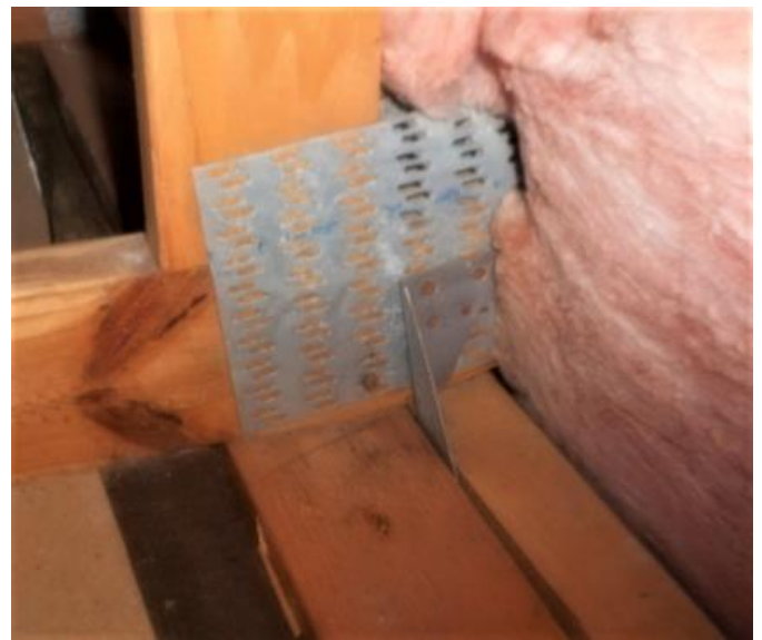
Truss Connection
