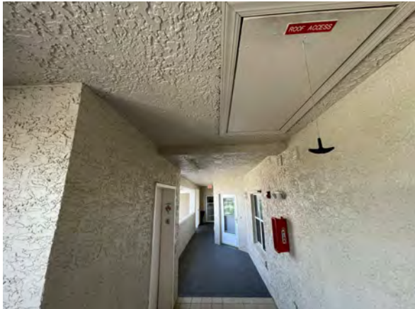
GENERAL VIEW OF BUILDING EXTERIOR FINISHES
