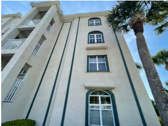
GENERAL VIEW OF BUILDING EXTERIOR FINISHES
