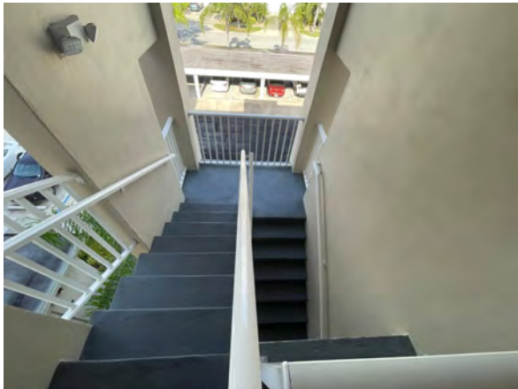
GENERAL VIEW OF STAIRWAY
