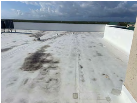
GENERAL VIEW OF TYPICAL ROOFTOP
