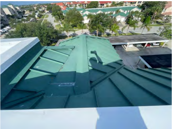
GENERAL VIEW OF TYPICAL ROOFTOP
