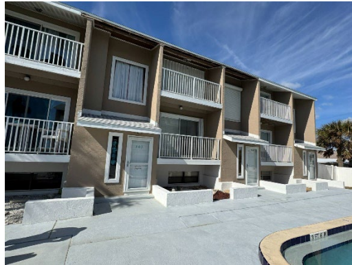
General View of the Property
