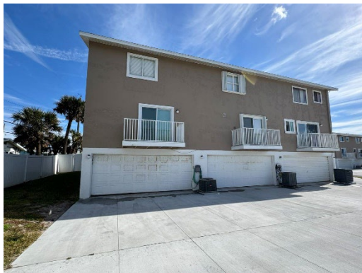
General View of the Property
