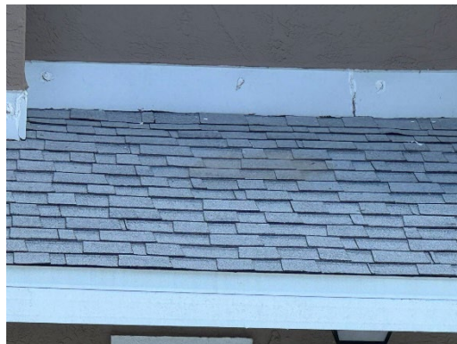
General View of Rooftop
