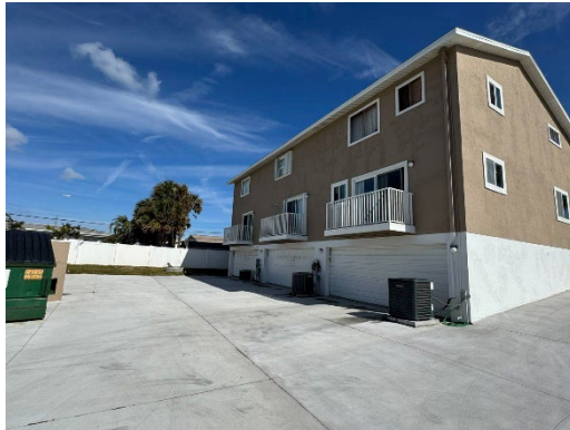
General View of the Property
