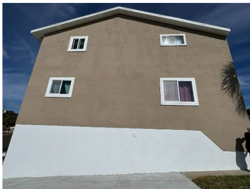
General View of the Property
