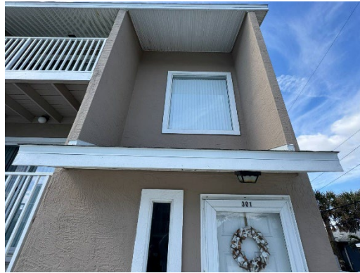
View of Typical Unit Window
