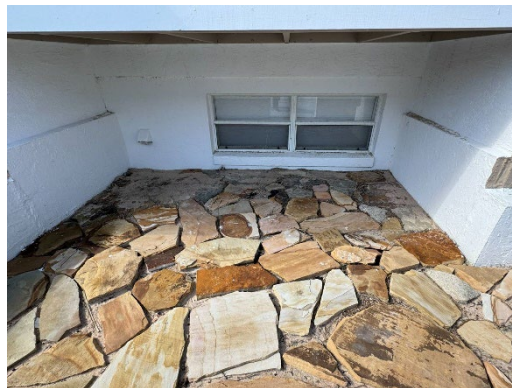
View of Typical Unit Window
