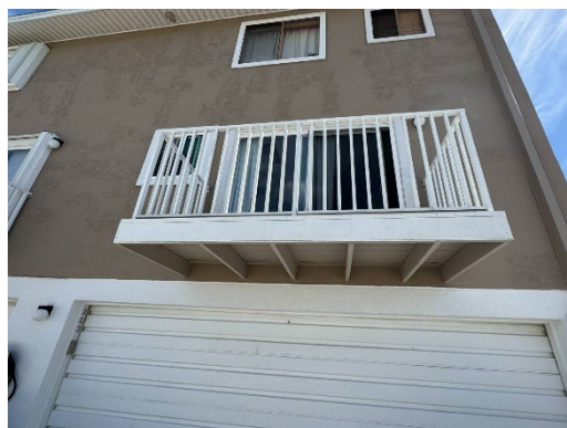
View of Typical Balcony
