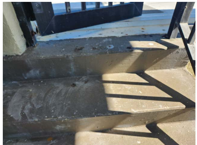
CONCRETE ROOF DECK
