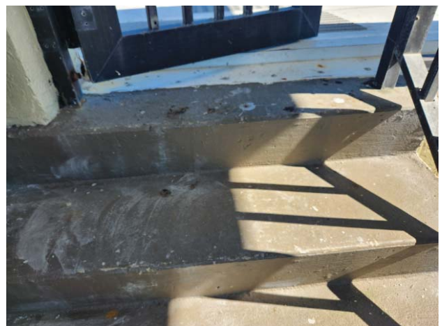
CONCRETE ROOF DECK
