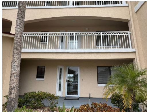
GENERAL VIEW OF GUARDRAILS
