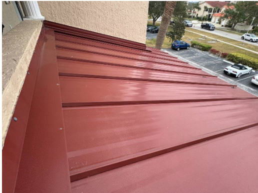
GENERAL VIEW OF TYPICAL ROOF
