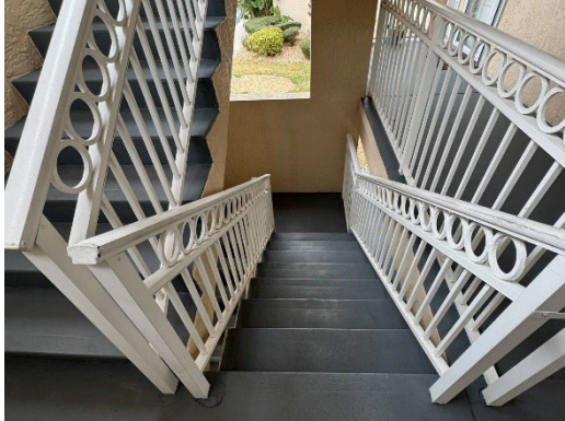
GENERAL VIEW OF TYPICAL STAIRWAY
