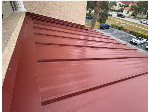
GENERAL VIEW OF TYPICAL ROOF
