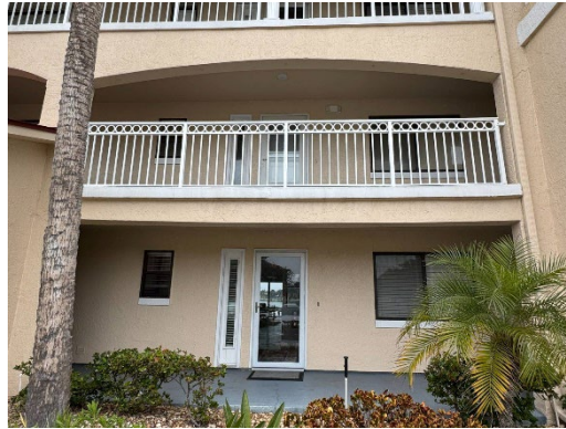
GENERAL VIEW OF GUARDRAILS
