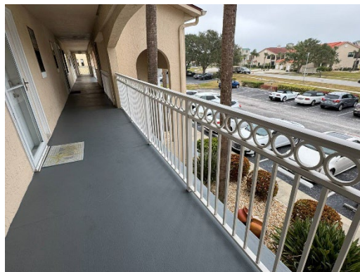
GENERAL VIEW OF TYPICAL ELEVATED WALKWAY
