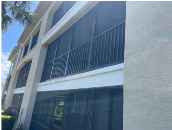
GENERAL VIEW OF BUILDING
