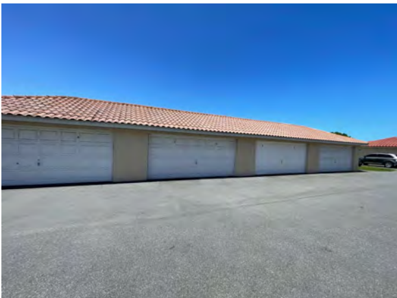
GENERAL VIEW OF PARKING
