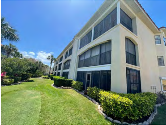
GENERAL VIEW OF BUILDING
