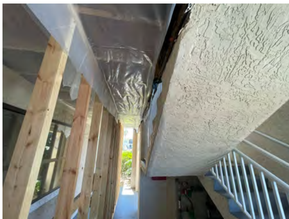
REPAIRS IN PROGRESS
