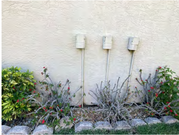
VIEW OF BUILDING FINISH
