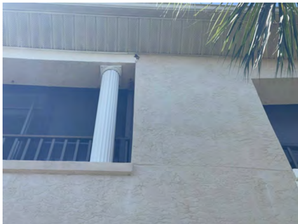
VIEW OF BUILDING FINISH
