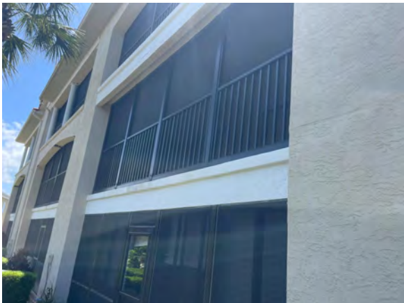
GENERAL VIEW OF BALCONIES AND REAR OF BUILDING
