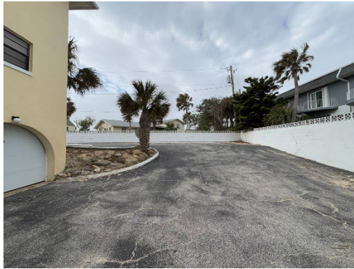
View of Driveway
