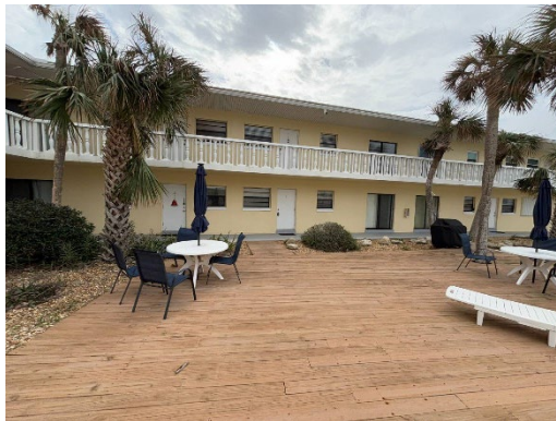
General View of Deck
