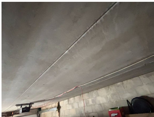
General View of Concrete Slabs and CMU Walls
