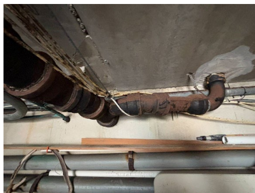
View of Drain Line
