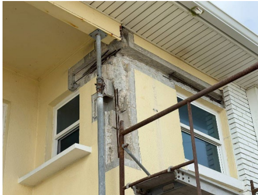
General View of Current Restorations
