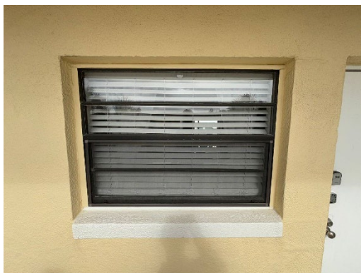
View of Common Area Windows/Doors
