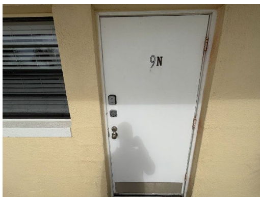
View of Common Area Windows/Doors
