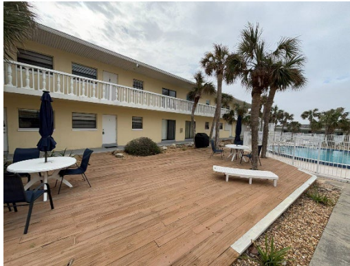
View of Typical Elevated Walkway
