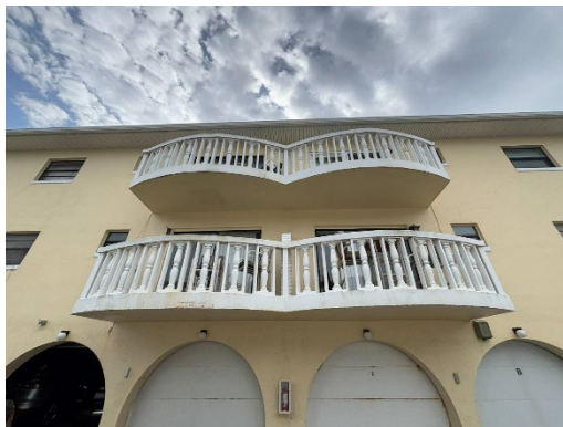
View of Typical Balcony
