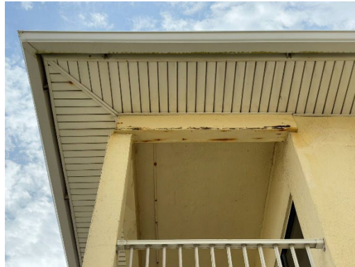
General View of Soffit
