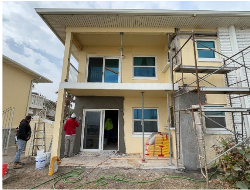
General View of Current Restorations
