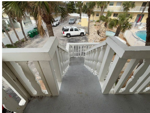
View of Typical Staircase
